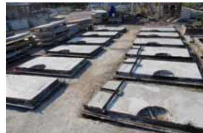
Construction of pre-cast slabs for 'mark3' VIP latrines for distribution in Ugu Municipality
