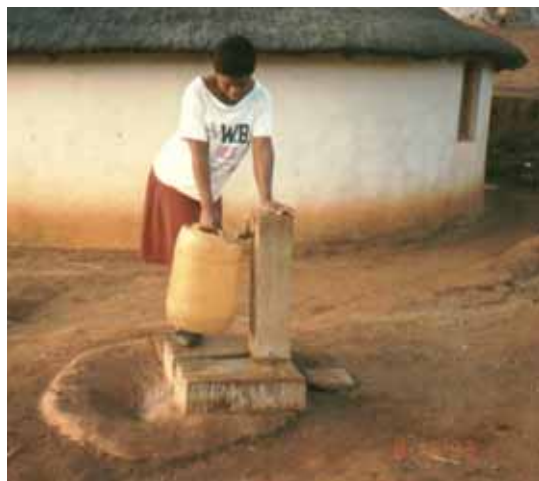
Tap stand in the KwaNyuswa ward of Ndwedwe near Verulam. The project was built entirely by the community. Note the way a drain has been built for the waste water, which led away to a garden, the builder's own initiative.
