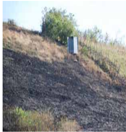
Latrine location on a slope with minimal lining of pit can result in contamination of downslope soil and garden produce.
