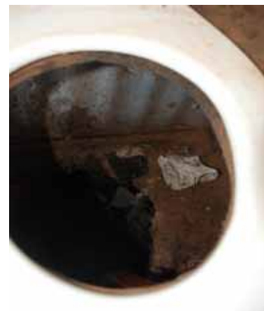
Poor slab design leading to misdirected faecal collection (alias the 'poopcatcher' syndrome)
