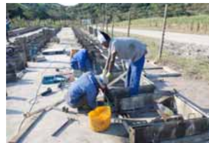
Construction of pre-cast slabs for 'mark3' VIP latrines for distribution in Ugu Municipality
