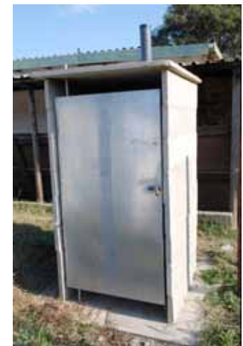
Mark3 (above) and mark2 in use in KZN. Note swivel steel door on new version.
