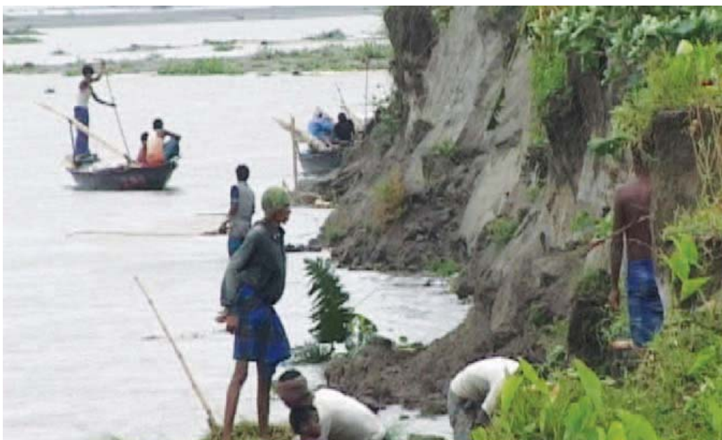
River Erosion (Source: PPA Field Study)
